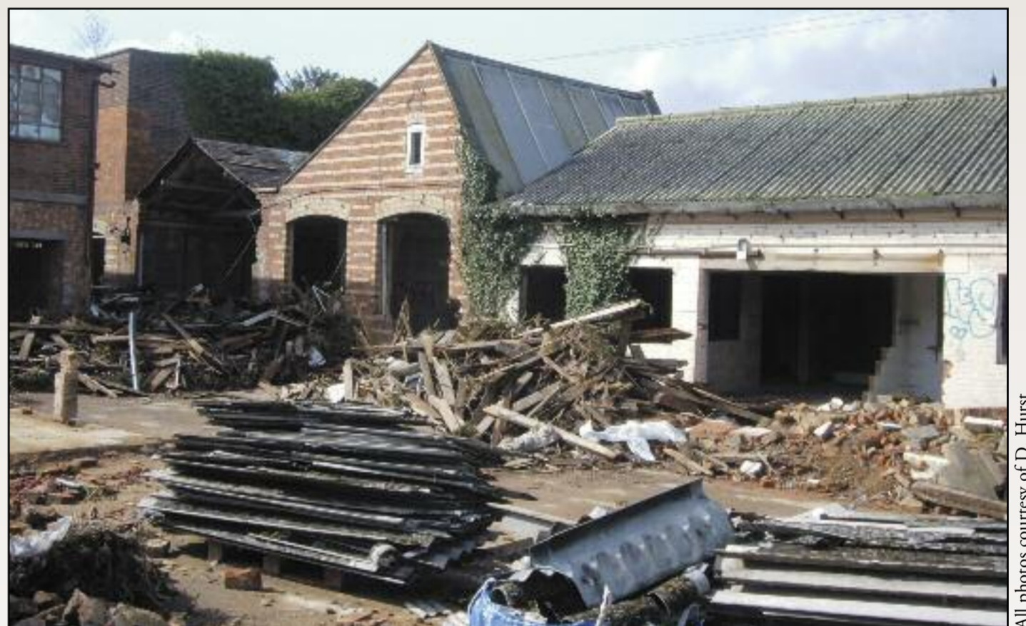
Demolition of the factory
