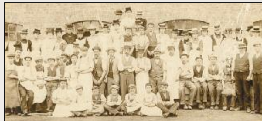
Roots workers at Tavistock Street works
