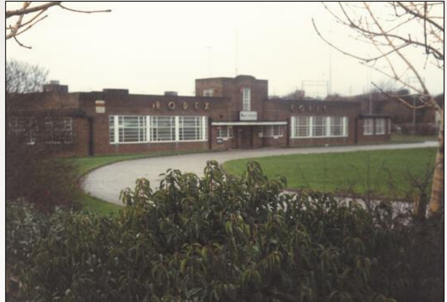
Rodex Coats building. January 1990
