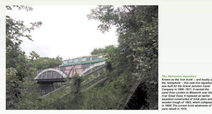
The Wolverton Aqueduct Known as the 'iron trunk' - and locally as the 'ackeyduck' - this cast iron aqueduct was built for the Grand Junction Canal Company in 1809 -1811. It carried the canal from London to Blisworth over the river Great Ouse. It replaced an earlier aqueduct constructed of brick piers and a wooden trough of 1803, which collapsed
