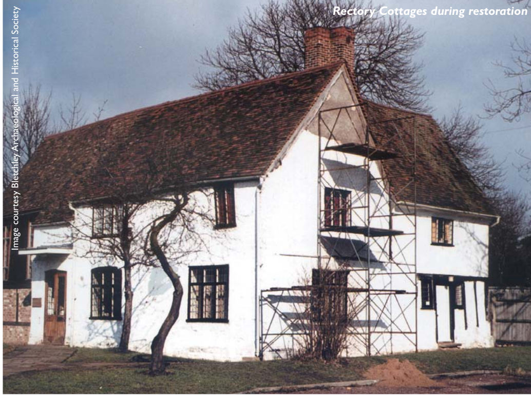
Rectory Cottages during restoration
