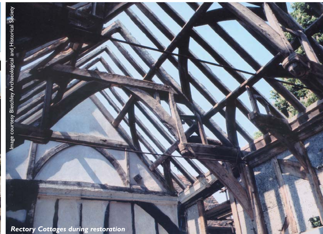
Rectory Cottages during restoration
