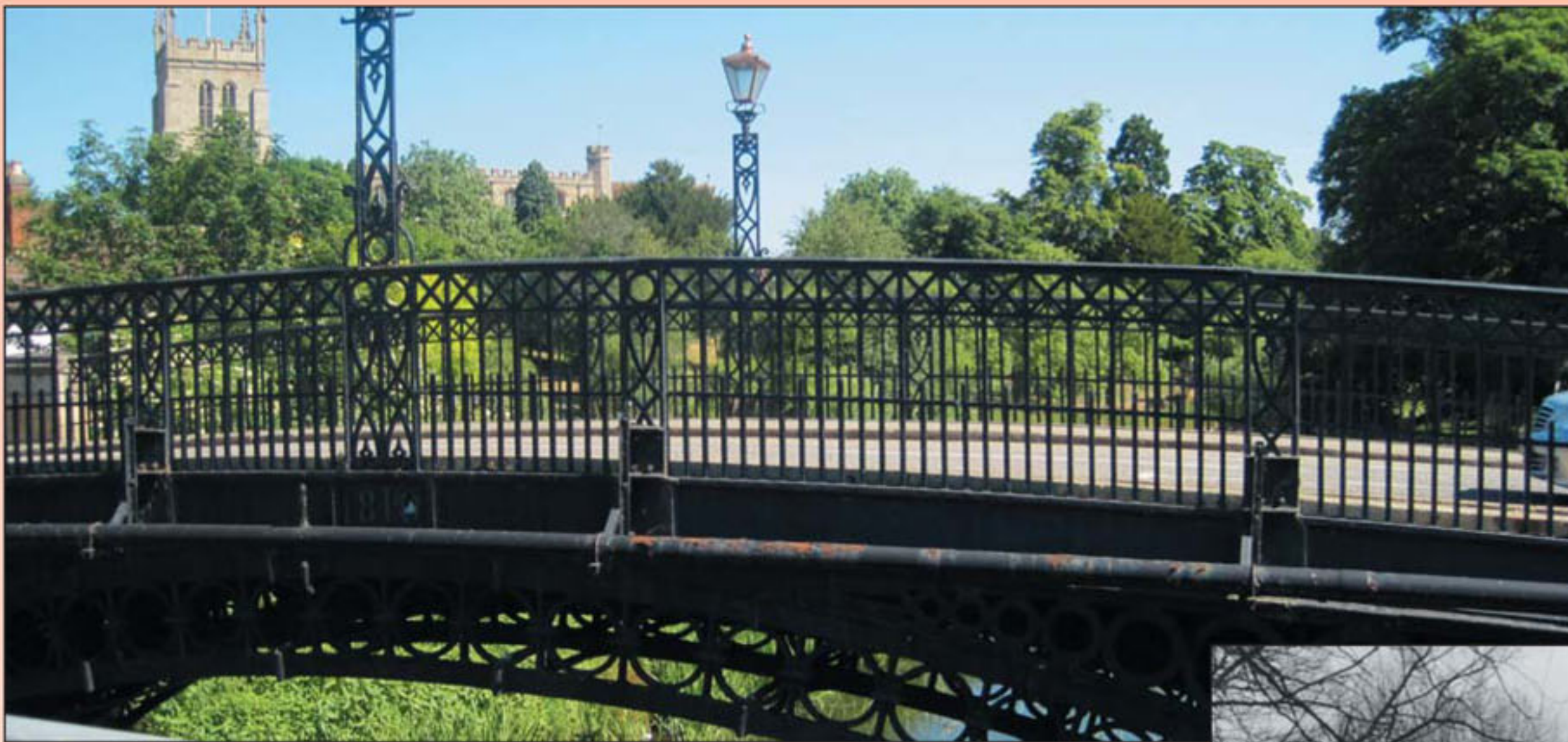
Tickford Bridge June 2010
