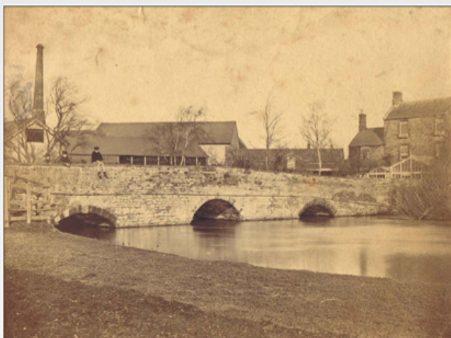
The east side of the pre 1894 old 'Duchy' bridge at Olney.
