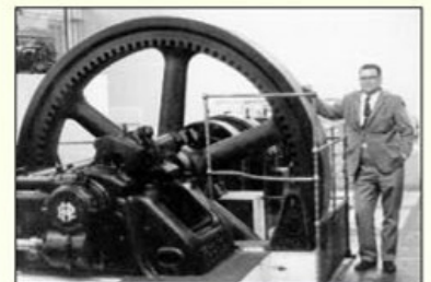
Flywheel at Fenny Stratford Repeater Station
