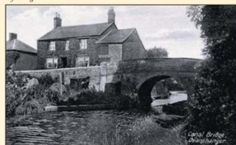
Wharf House, Canwin's Wharf, showing the hump-backed bridge which was demolished in 1972
