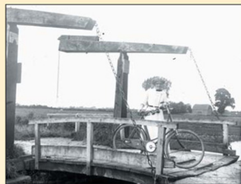
Lift bridge circa 1910
