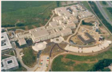
The hospital under construction
